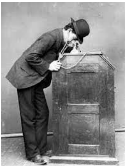
The Kinetophone (earphones lead to a phonograph in the cabinet)
